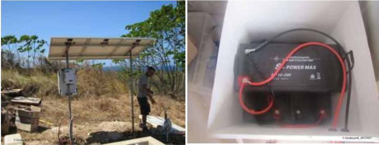
**Figure :** The left photo shows the technician's working during the installation and the right photo shows the three (3) batteries installed in the basement.
