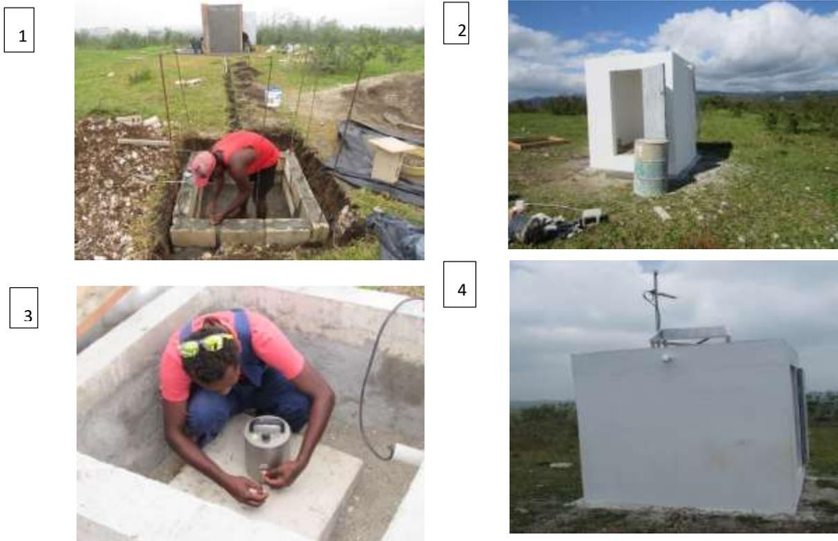
*The different steps in the installation of the MKV seismograph from 29 June to 10 July 2015 beginning with the construction of the SHED foundation (1) the finishing of the shed (2), the installation of the equipment (3) and the installation of the data transmission system (4)*
