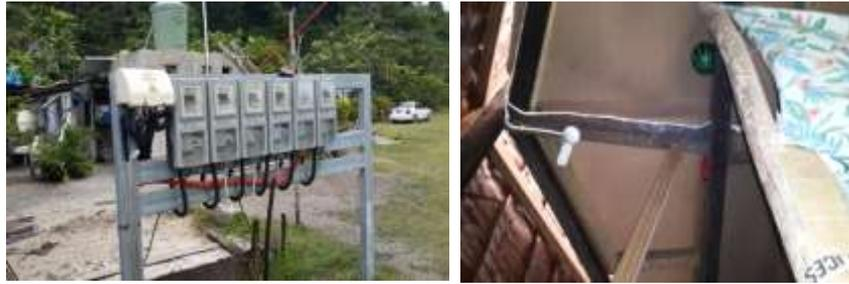
Photo: Picture on your left depicting a series of prepaid meters with 5 amps installed for small domestic customers in Siviri Village, North Efate. On your right, a photo featuring a light bulb in a small traditional house as part of house wiring that consist of 2 light bulbs, 2 power outlets and two switches.
