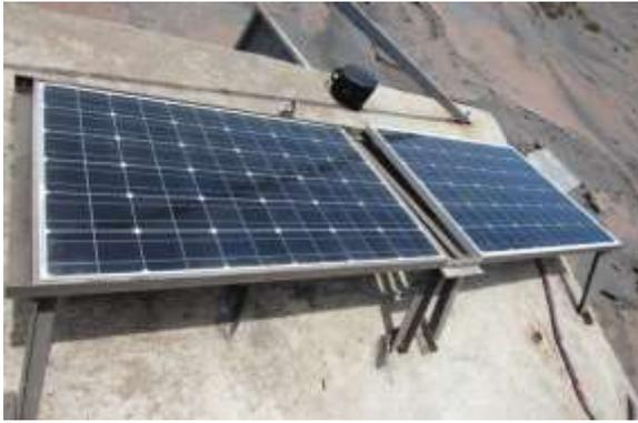
*Solar panels of 140W installed on the shed*
