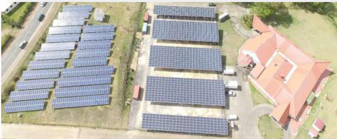
Photo: Aerial view of the 645 kWp solar installation at the Parliament area
